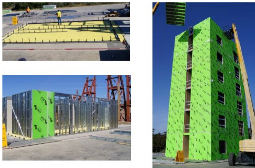
Figure 34. CFS-HUD test building on the world's largest outdoor shake table (LHPOST) at UCSD (photo credit: [32])
