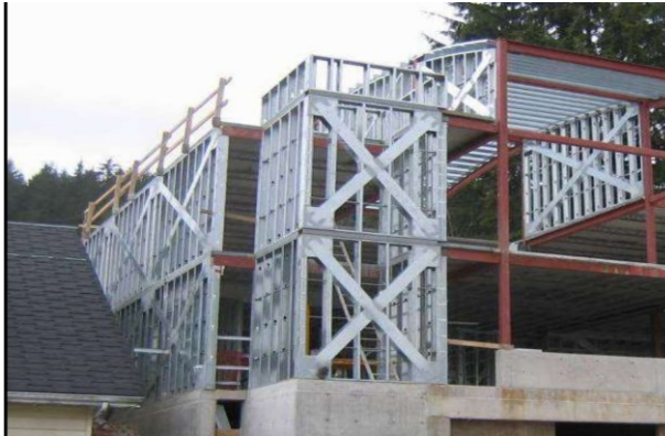
(c) strap-braced walls (image source: [5])
