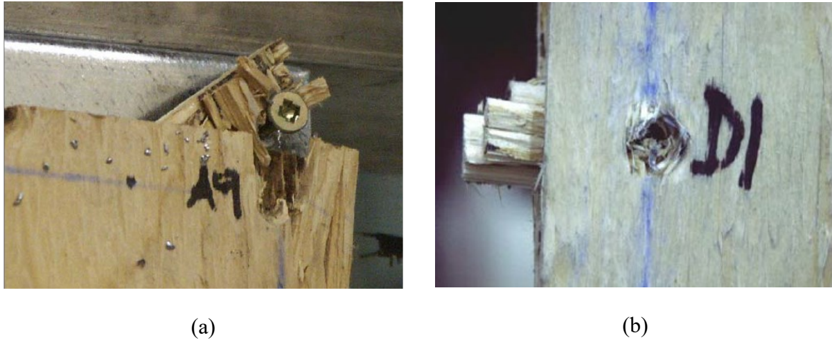
Figure 6. Examples of failure modes of walls with WSP sheathing: (a) sheathing tear-out at corners; (b) wood bearing failure (image source: [3])
