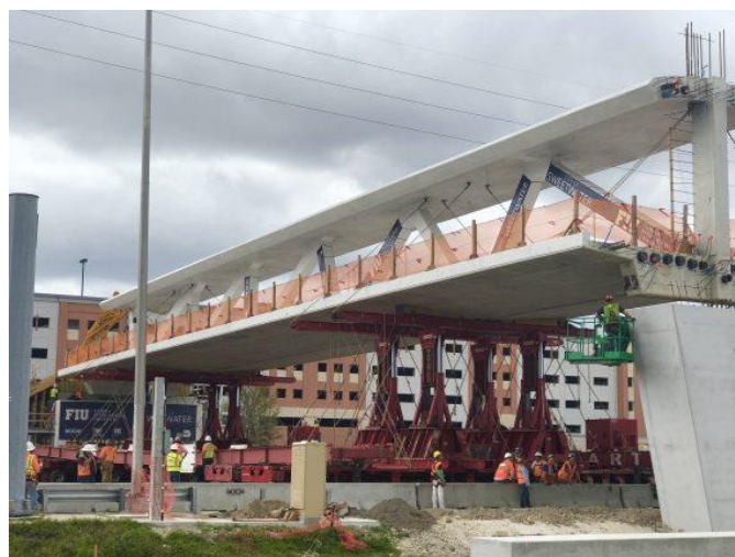
Fig.1 SPMT jacking truss bridge (2018)
