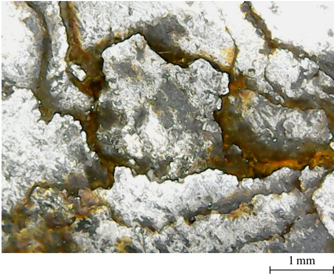
Figure 13: Image of cracked rail surface
