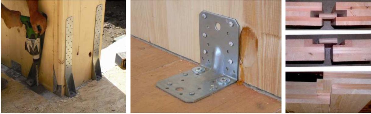
**Figure 1.** Hold-down, angle bracket and screwed-joints
