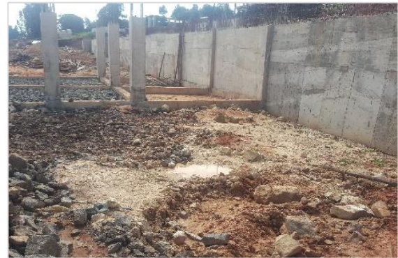
Fig. 5 Settlement and non-conforming backfill materials
