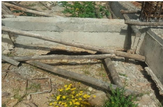
Fig. 5 Settlement and non-conforming backfill materials
