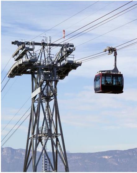
(a) Exemplary pylon structure of Ritten's cableway (South Tyrol, Italy), source: provinz.bz.it.
