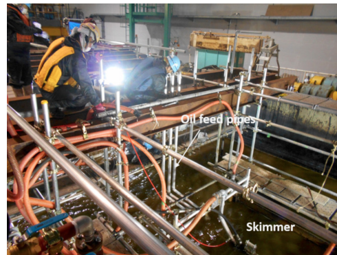
(b) Oil feed onto the water surface
