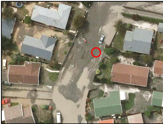
(c) Severe Liquefaction
