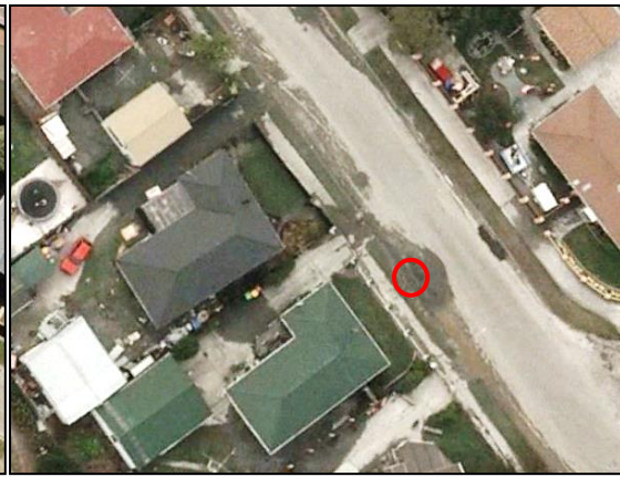
(b) Moderate Liquefaction
