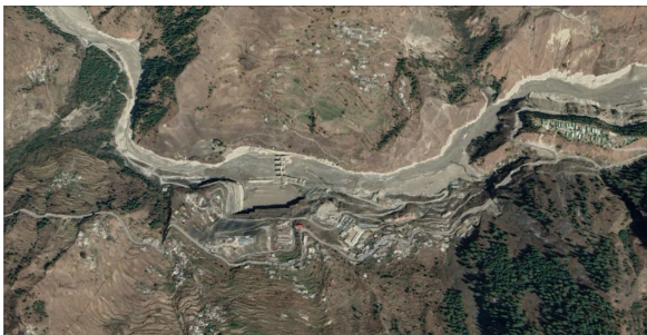
Figure 2: This map shows Tapovan Retreat, Uttarakhand, where several homes and shops are located, that is flooded after the Tapovan dam breaks.
