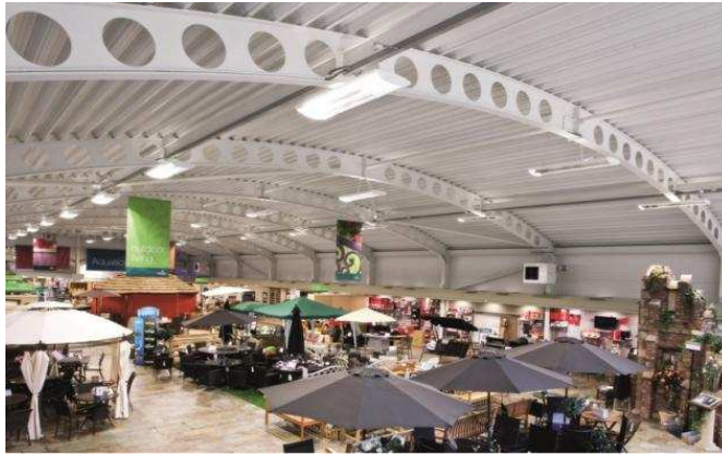
Figure 1. Circular shaped Reduced Web Sections incorporating services (SteelConstruction.info, Image courtesy of ASD Westok Ltd.).
