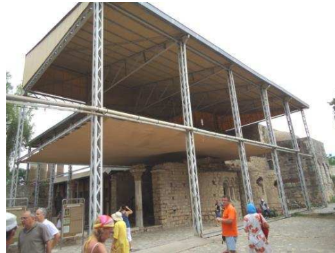
Figure 2: Protective cover above Saint Nicholas Church, Demre, Turkey (Ertosun [3])
