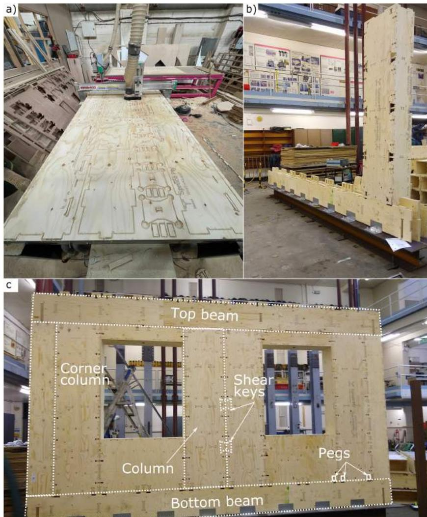
FIG. 2: Fabrication and assembly of the specimens: a) CNC cutting of the specimens, b) installation of the bottom beam and assembly of the first column, and c) final construction
