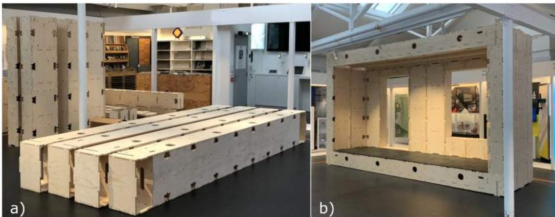
FIG. 1: Wikihouse Skylark installation at the Building Centre architectural gallery in London (UK): a) components and b) assembly. (Photo courtesy of Alastair Parvin)
