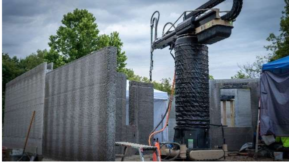
Figure 1 - Apis Cor's "Frank" robot is an example of the Fixed Base Radial Arm architecture (Photo courtesy of Apis Cor)
