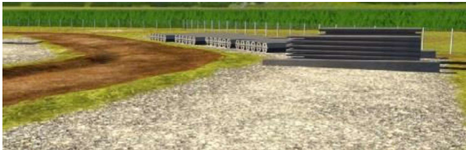
Figure 3. Precast concrete Hexcrete components at a tower site
