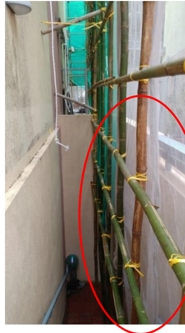
(d) Scaffold cutting along the staircase
