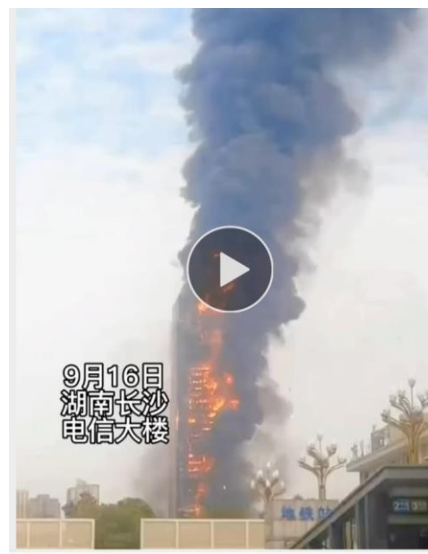
(“Fire at the China Telecom Building in Changsha, Hunan on 16 September 2022”. Video from WeChat. Channels (Kao Shan Tun Xian Hua))
