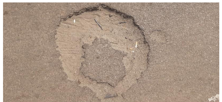
Figure 12: Pothole
