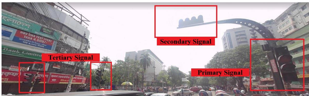
Figure 36: Traffic Signals at Panthapath Intersection Node
