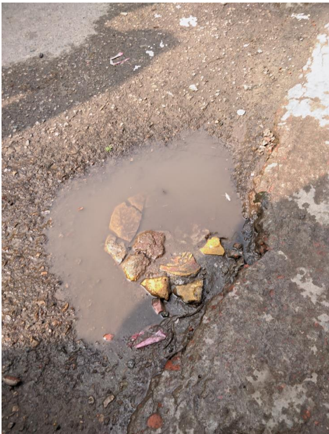
Figure 10: Pothole
