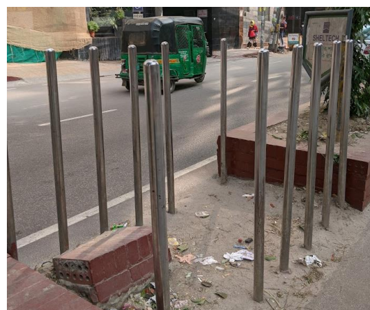
Figure 25: Median Opening with Vehicle Barring
