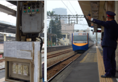
TRA's operating practices may be labour intensive, but resulting service quality is high: stationmasters' controls feature departure bells, schedule simplifiers, and "good to go" plungers (left); Hsinchu's stationmaster (right).
