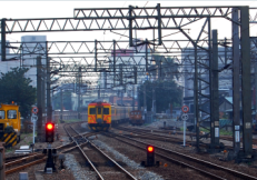
Train terminations and transfers occur at interchanges where double island platforms and full crossovers are provided. The Japanese Tokyo DR3000 DMU is departing from Shulin station, using crossovers for yard access.
