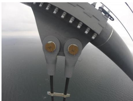
Figure 2 - Upper end of the hanger
