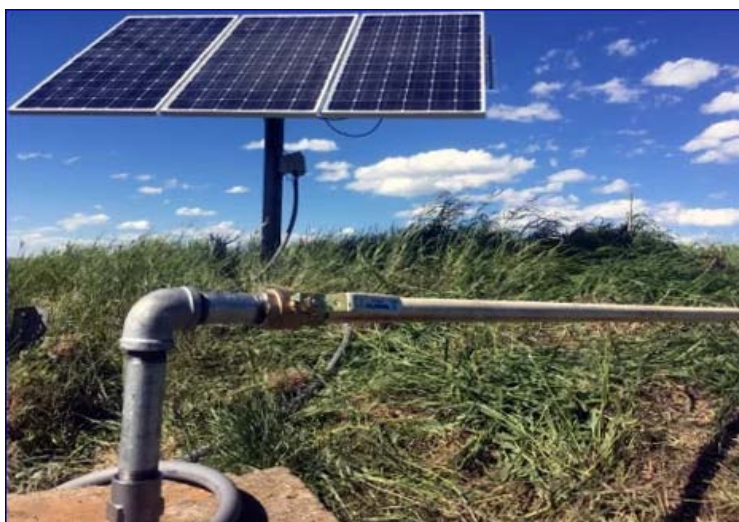
Figure 10. show atypical solar energy system for Agriculture[40]
