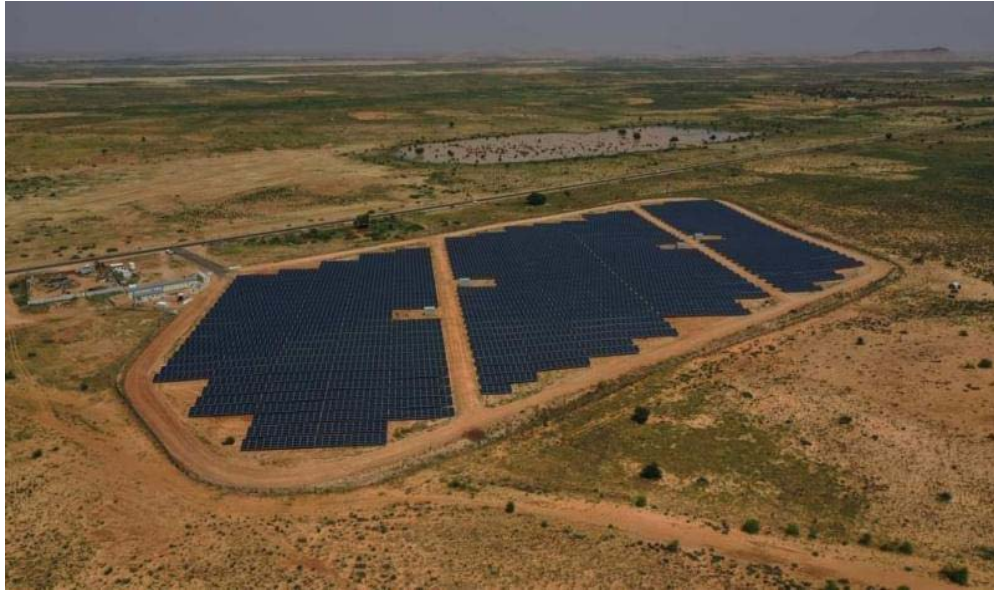
Figure 1. Example Solar panels of grid-Tied System/On-grid system of Elfashir Solar farm (5 MW Capacity Project)
