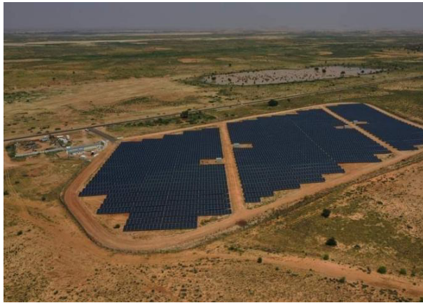
Figure 1. Example Solar panels of Grid-Tied System/On-grid system of Elfashir Solar farm (5 MW Capacity Project)
