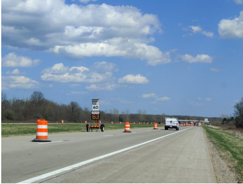
FIGURE 1. Speed feedback trailer positioned at the end of taper at WB I-69 work zone
