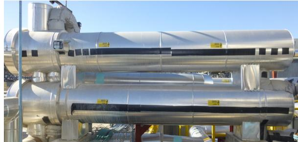
Figure 2: Two-unit multi-pass shell-and-tube heat exchanger
