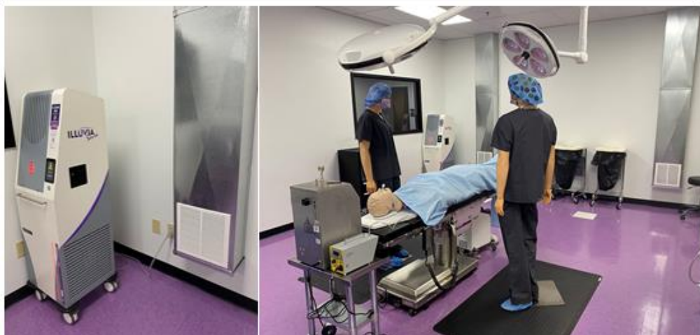
Figure 1: The configuration of the simulated OR is shown. Downward unidirectional airflow delivers HEPA filtered air at the center of the room. Near each corner of the room are return air ducts. The
