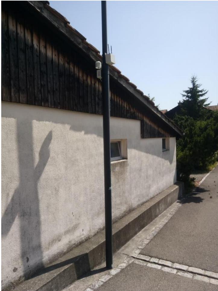
Figure S 4-9: ambient temperature and humidity sensor mounted at a lamp pole (backside).
