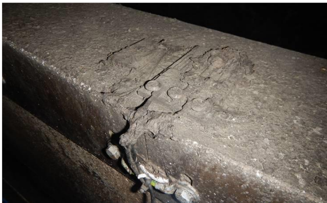
Figure S 9-4, left: Capacitive sensor for overflow discharge detection at the weir crest basin RUB 59 after three years of operation. Photo: S. Bloem, Eawag. Right: Cross-section through overflow structure (not drawn to scale), including inflow chamber (2), retention tank (1), overflow to receiving water (3) and US level sensor (h01) and the capacitive sensors (bm332 and dl311).
