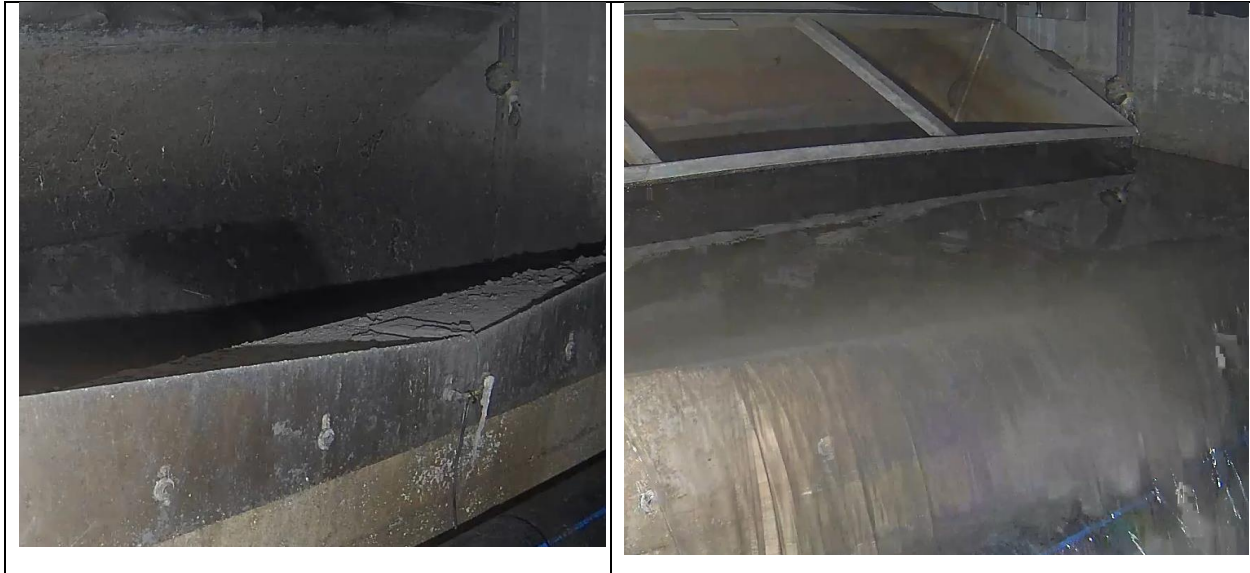
Figure S 4-4 left: the Decagon sensor, i.e. Meter 5TM mounted on a weir crest in dry environment; right: submerged sensor in case of an overflow event.
