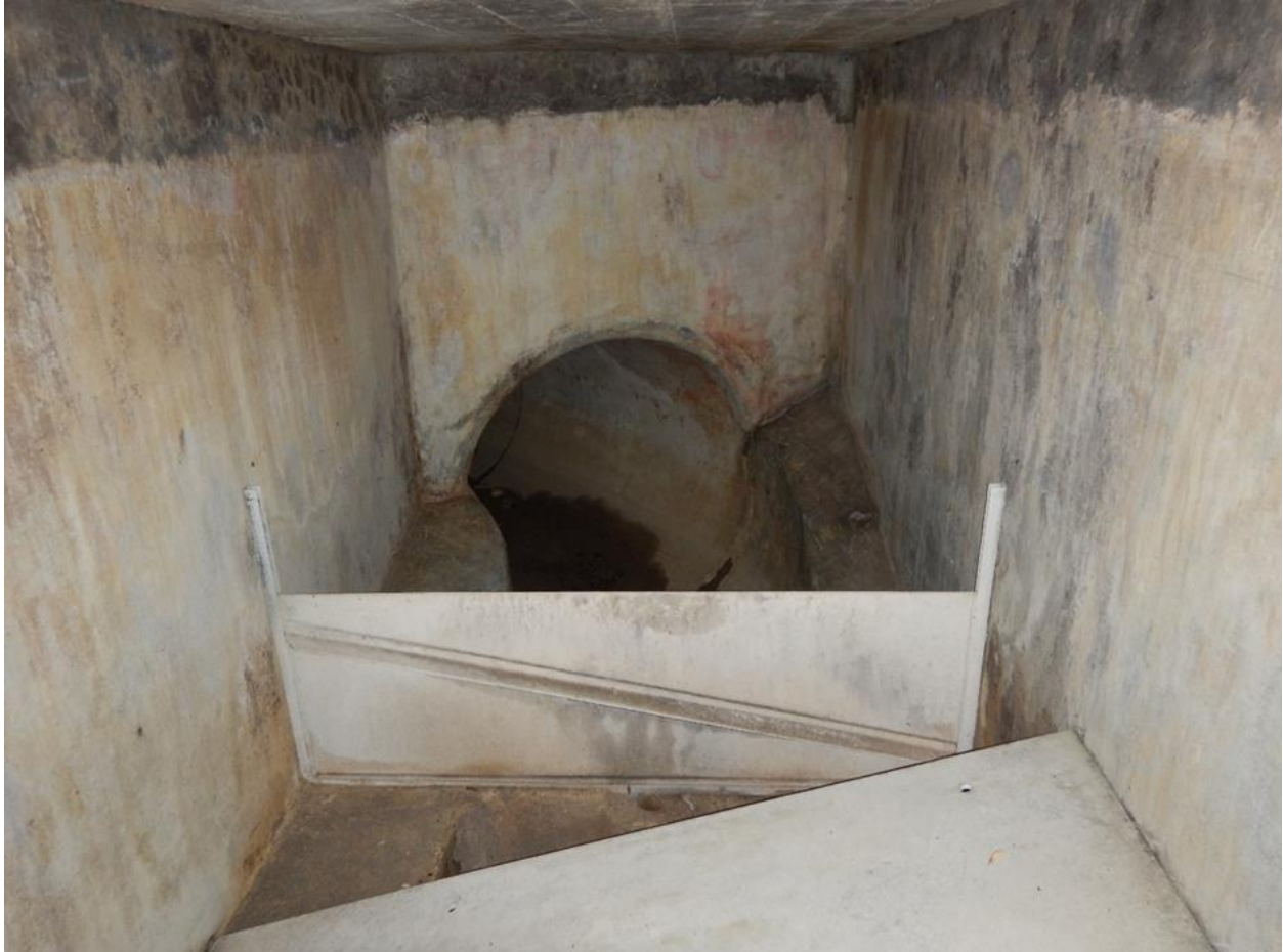
Figure S 3-11 stormwater overflow RU 48b , which is considered inactive under given circumstances.
