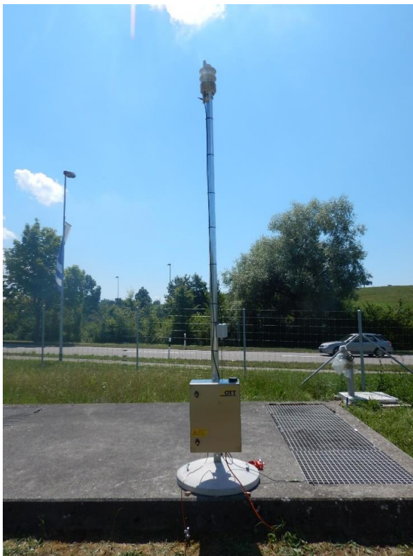
Figure S 4-13: WS-700 on post with concrete base.
