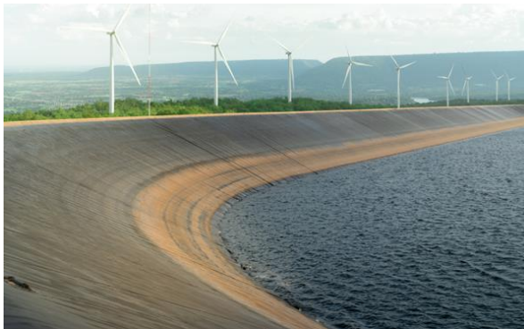
3 Geomembrane in a pond application. Free Stock Media. (Fahroni, 2023)
