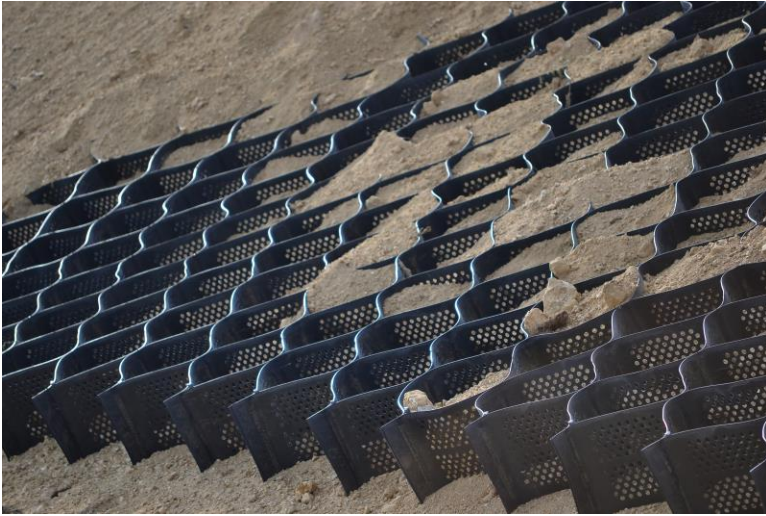
Figure 13. Geocells filled with sand. Free Stock Media. (Alecsps, 2023)
