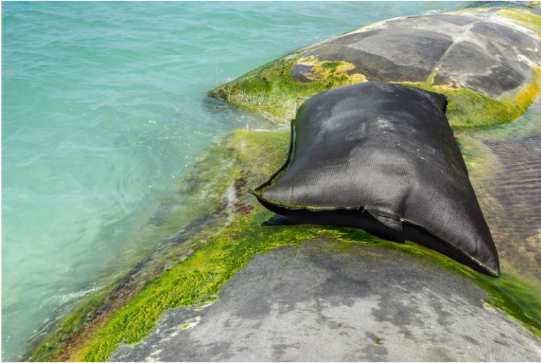
Figure 14. Geotubes in a coastal engineering project. Free Stock Media. (Gouida, 2023)
