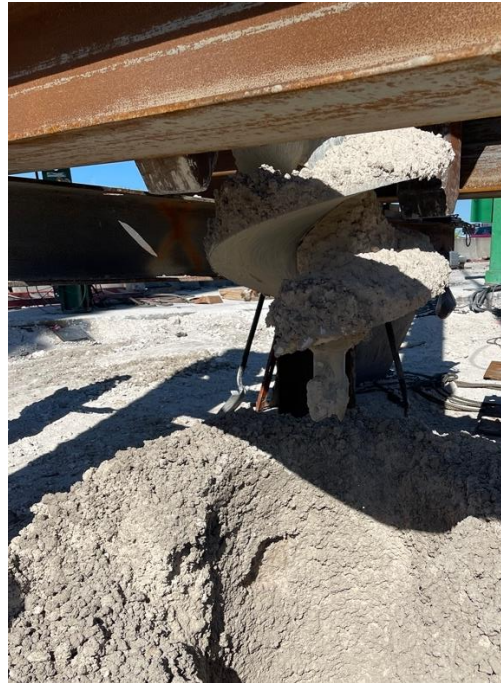
Figure 7. Excavated soil in Downtown Miami area.
