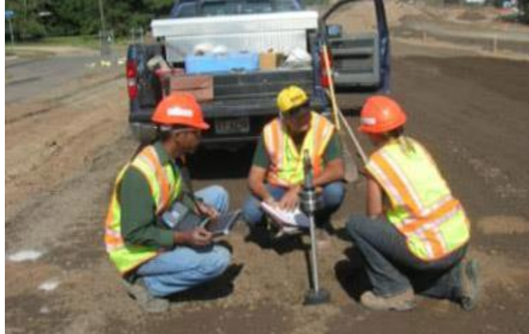
Figure 10. Technicians Check during compaction. Public Domain Media.
