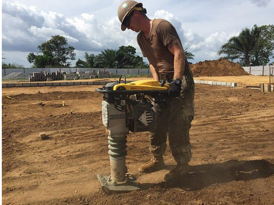
Figure 13. Manual Tamping. Public Domain Media.
