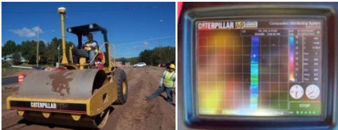
Figure 5. Intelligent Compaction Roller and Compaction Display. Public Domain Media.
