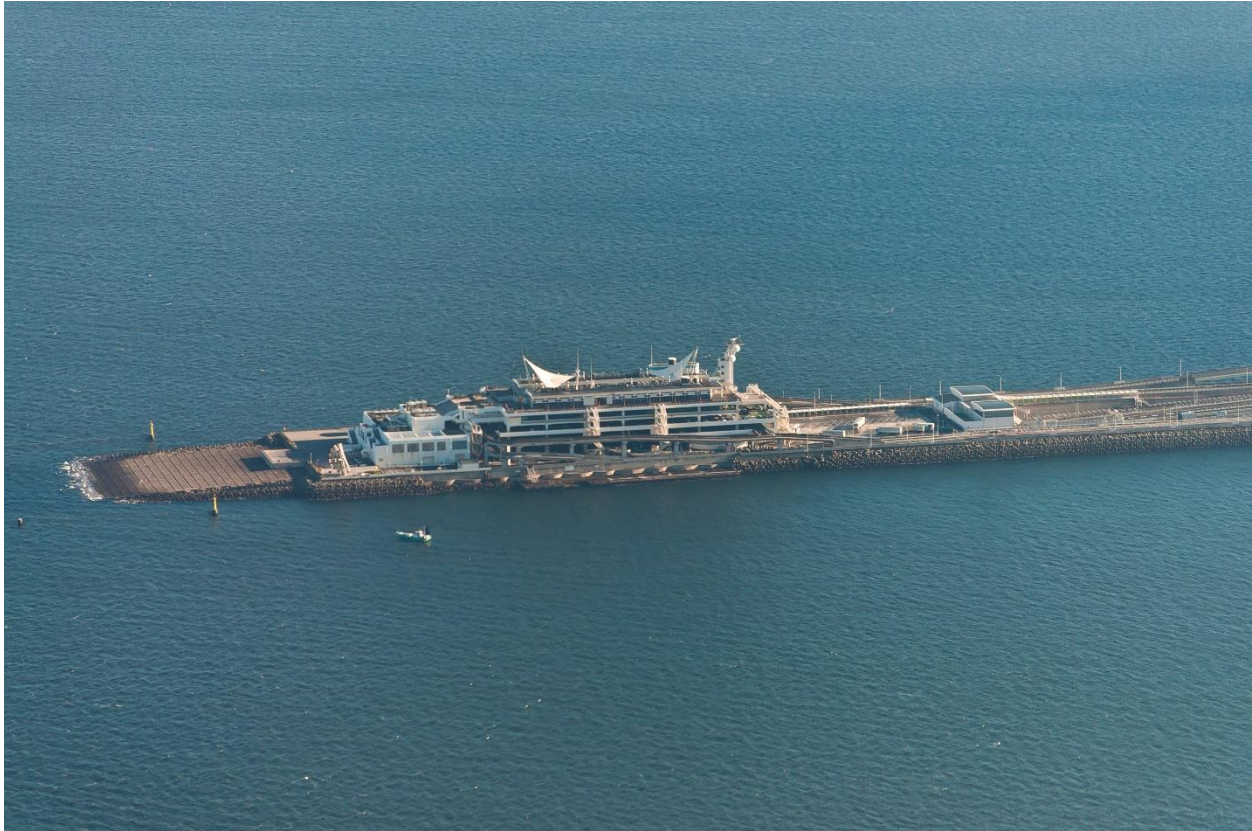
Figure 3. Tokyo Bay Aqua-Line Tunnel. Image by Chihaya Sta.
