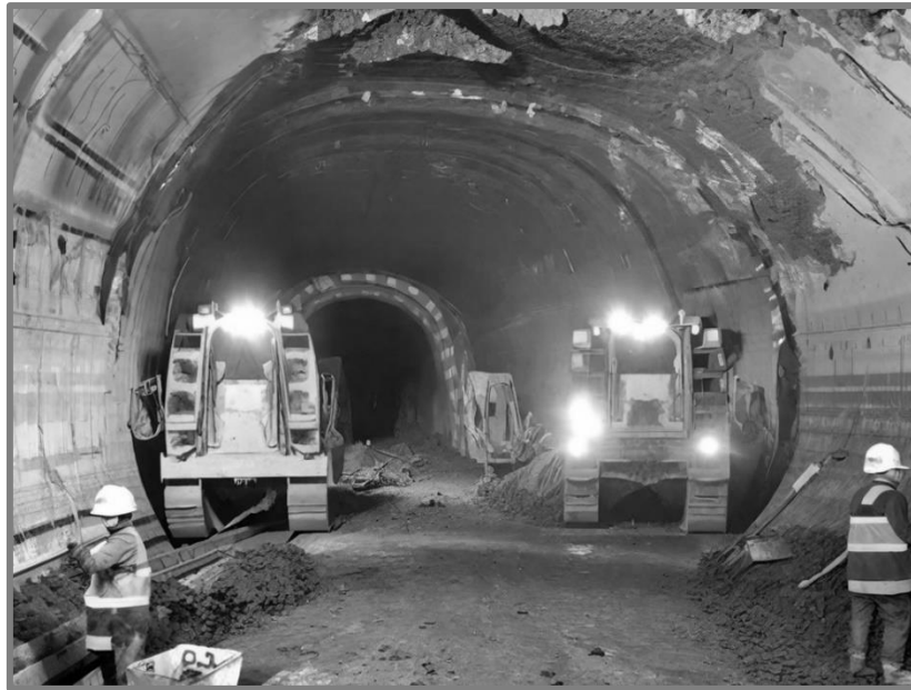
Figure 7.2. Construction of the Japan's Shinkansen
