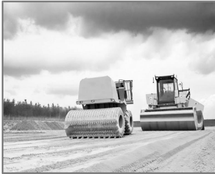
Figure 4.2. Padfoot Roller and Smooth Wheeled Roller in the Field
