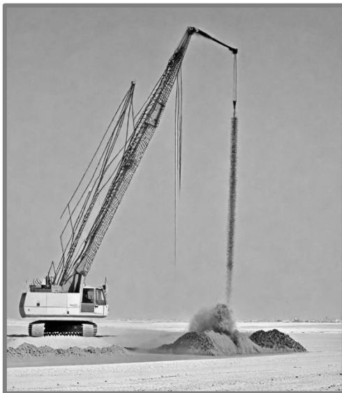
Figures 5.2 & 5.3. Deep Dynamic Compaction and Vibro-compaction Machinery
