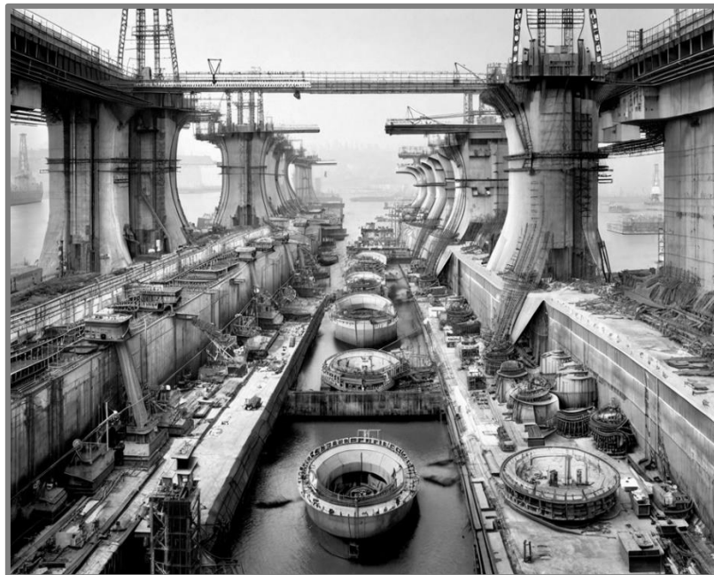
Figure 7.5. Construction of Three Gorges Dam
