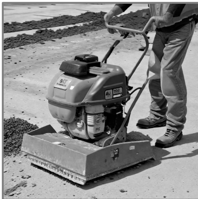
Figure 4.3. Plate Compactor utilized in the Field
