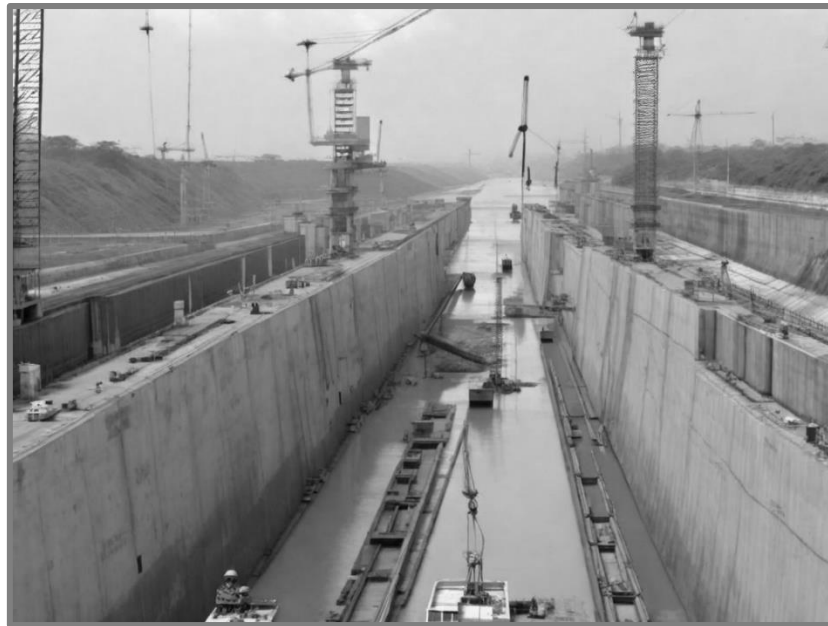
Figure 7.1. Construction of the Panama Canal
