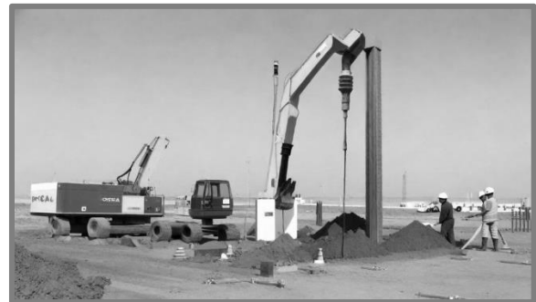
Figures 5.2 & 5.3. Deep Dynamic Compaction and Vibro-compaction Machinery
