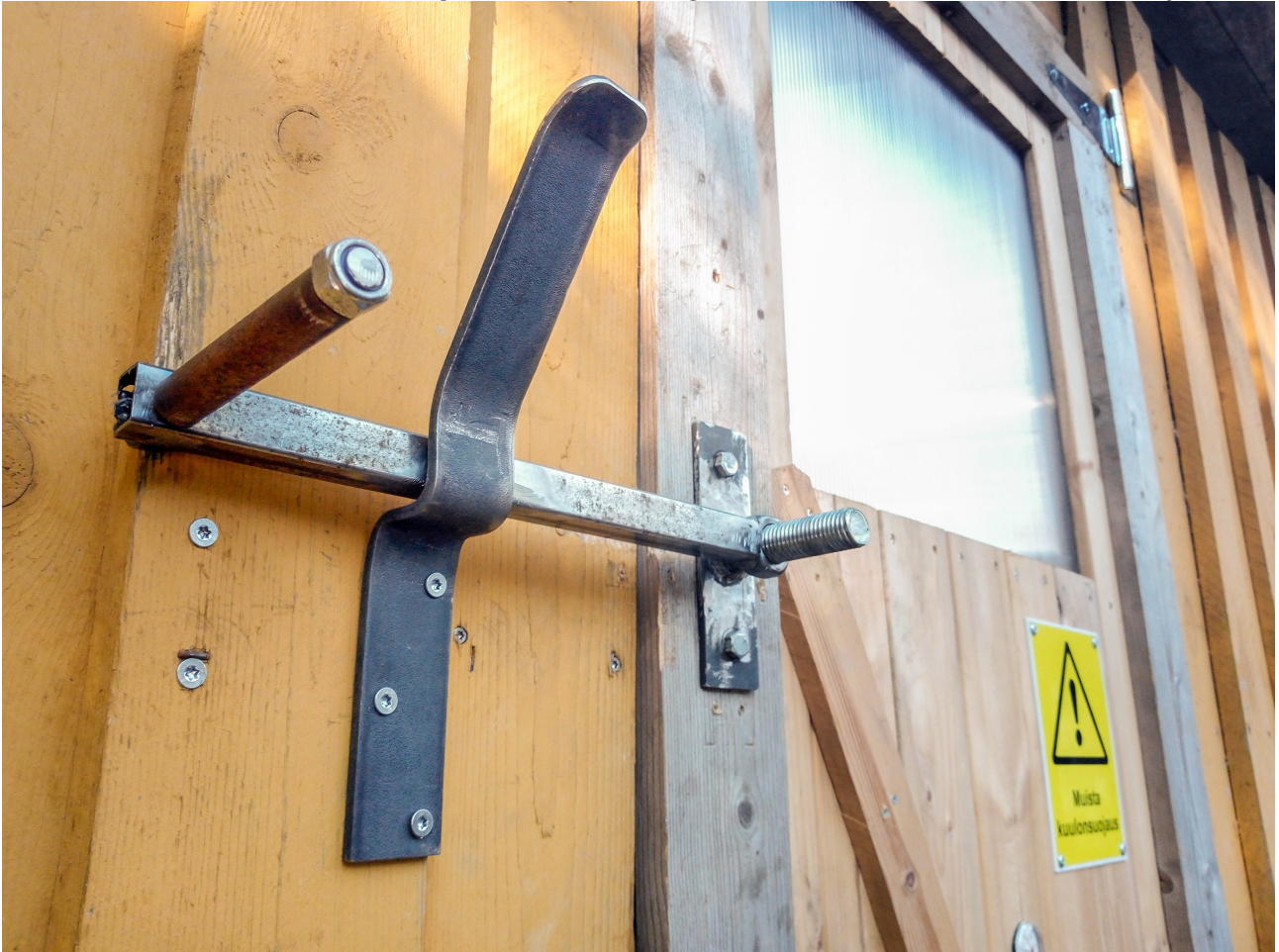
Figure 7. The new closing mechanism which was promptly invented using the EIDeM. The embodiment was done immediately, as the door became unexpectedly difficult to close after the earlier gaskets were replaced to thicker ones in a freezing and dark evening. The threaded rod, which is greased to avoid jamming, works as a rotation axis for the handle, and is also used to adjust how far the door is pushed during the sealing
