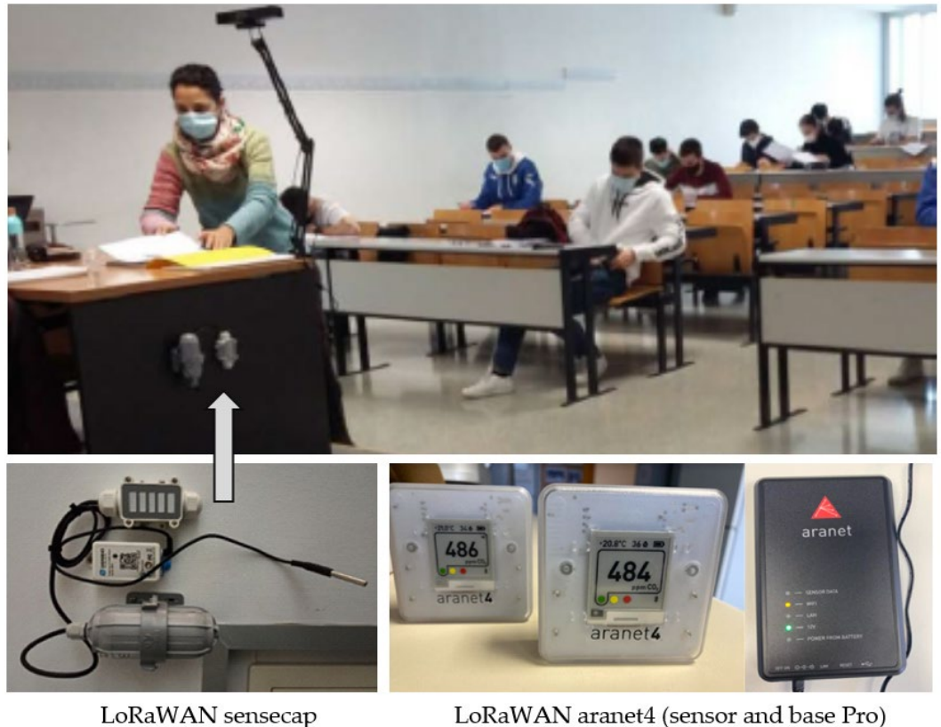
Figure 6. Sensecap [32] and Aranet [33] LoRaWAN sensors and their real installation in sensoriZAR .
