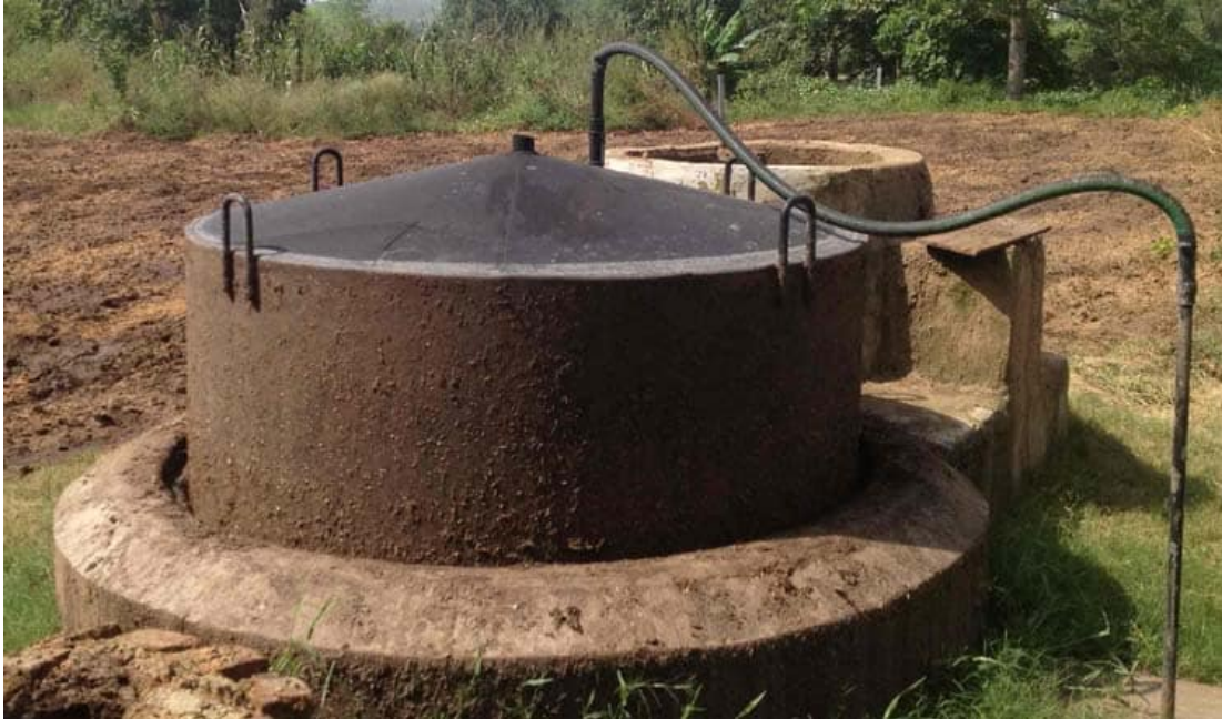
Figure 7.4: Floating cover digester in work.
