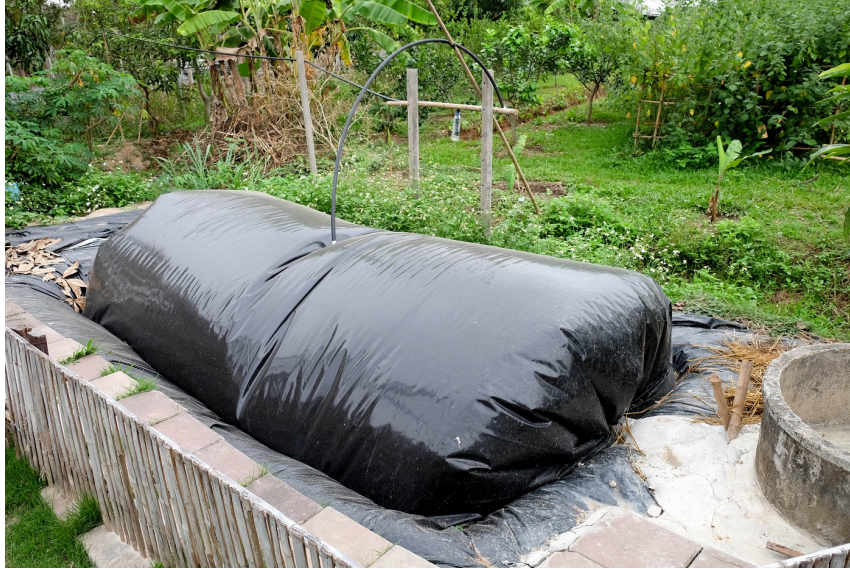
Figure 7.8: Plastic-tubular cover digester in work.
