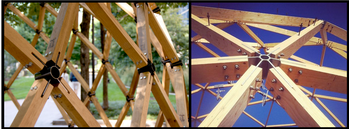
Figure 1: Splice node-connection “POLO-1” [9, 10].
