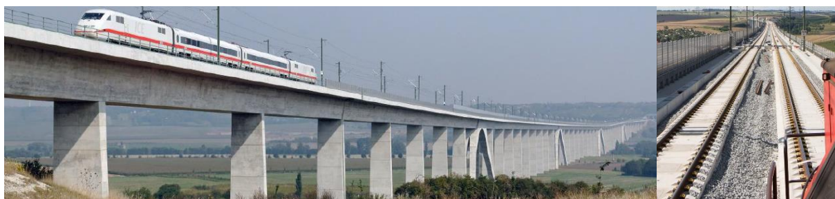
Figure 2: Photograph of the Unstrut Viaduct
