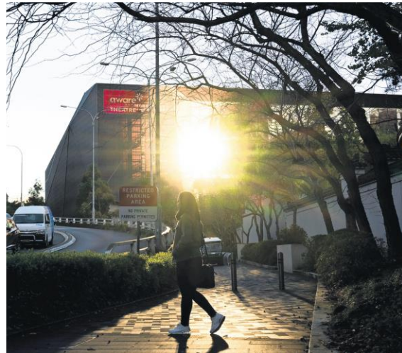
Fig. 2 – Winter solstice morning solar reflection off Theatre east facade glazing - photograph courtesy Sydney Morning Herald.
