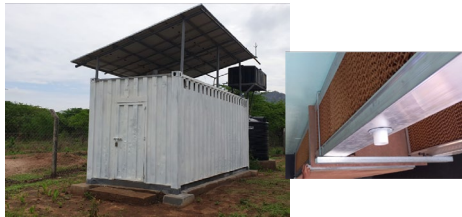
Figure 6. Images and schematics of various active cooling technologies (figures with credits from (a) ColdHubs, (b) Leap Energy and Smart Villages, (c) Thijs Defraeye, (d) Stephen Nyamai (an off-grid forced air evaporative cooling chamber near Kibwezi, Kenya) and Mahavir Acharya (evaporative cooling pads installed in the ceiling of a forced air evaporative cooling chamber near Bhuj, India) from https://www.cooling-chamber.mit.edu/ , (e) Village Infrastructure Angels (Efficiency for Access, 2021), (f) Amped Innovation 2024 ( https://www.ampedinnovation.com/products-solar-freezers )).
