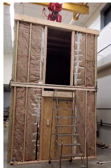
Figure 8: Enclosure for acoustics testing, FastFloor prototype at mid-height of specimen, testing conducted on floor
