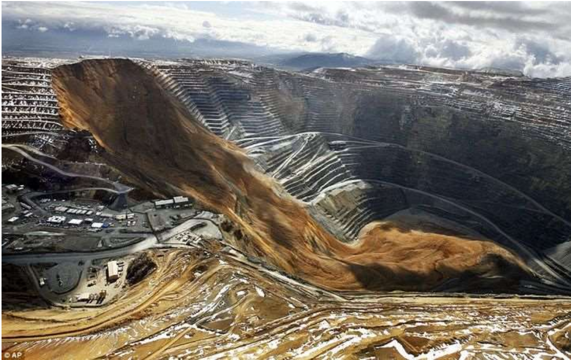
Fig. 1. The collapse of the side in the Bingham Canyon quarry (USA)
