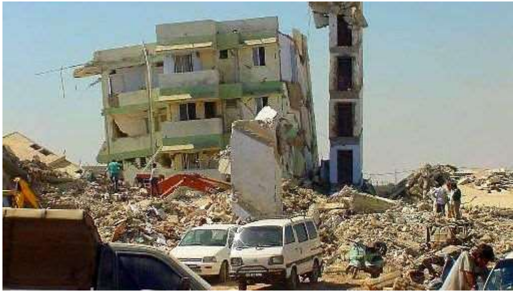
Figure 5:Gujarat Earthquake, India (2001)
