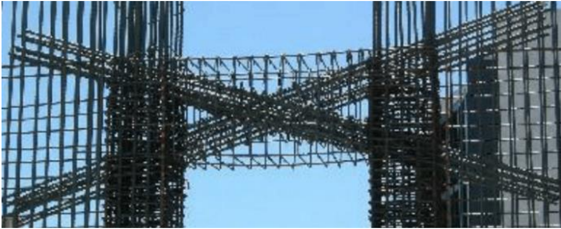
Figure (1-2): Diagonal reinforcement in coupling beams [3]
