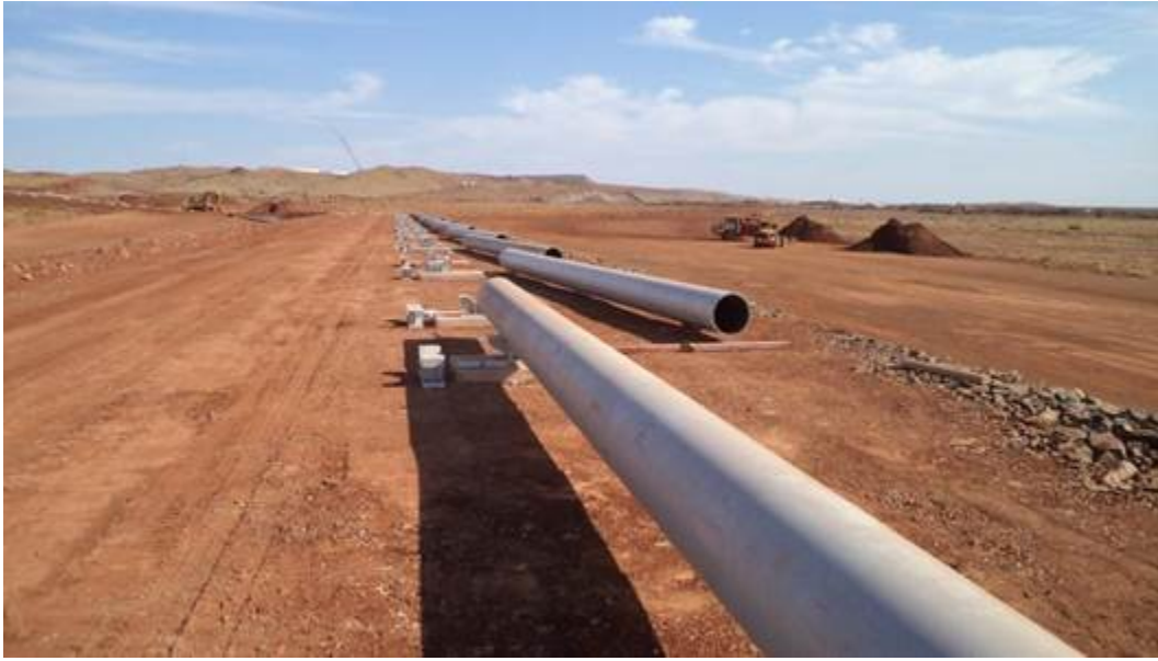
Figure 1: A long-distance slurry pipeline during its construction phase
