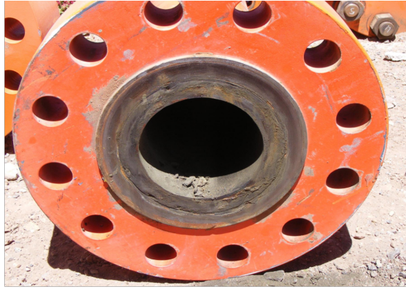
Figure 16: High-density polyethylene (HDPE) liner installation in copper concentrate pipeline. The inner ring consists of an HDPE stub end, tightly fitted into the steel, pressure-rated pipe.
