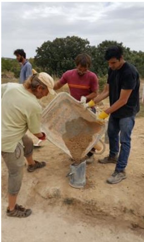
Fig. 8. Delivering mixture to the dome area.
