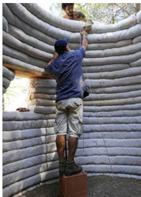
Fig. 10. Measuring correct distance of the ring edge with the central compass.
