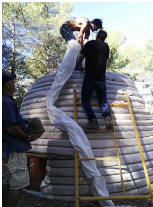
Fig. 9. Helping the placer of the sack. The dome team.
