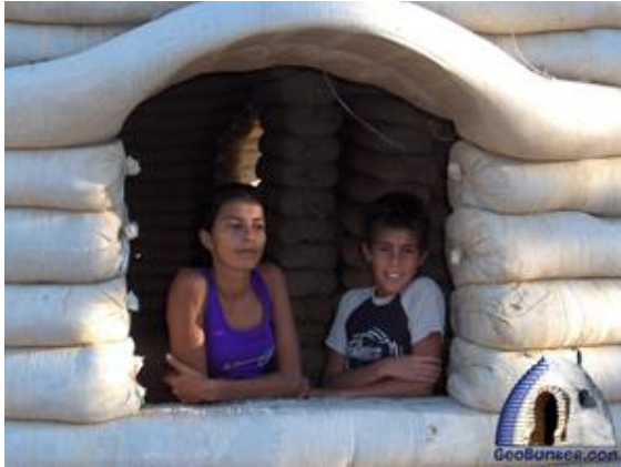
Fig. 17. Window opening after removal of the mold. Notice the self-sustainable arch form of the window according to the steps described above.
