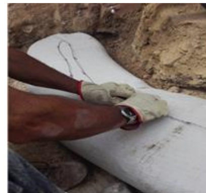
Fig. 13. Stitching barbed wire to the ring.
