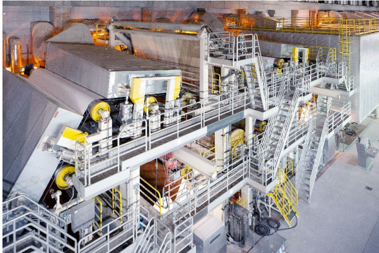
Figure 1 Stainless steel walkways, platforms, floors and supports at a paper mill.
