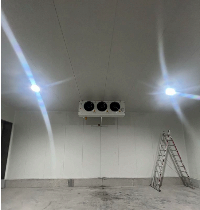
Figure 2a) New pre-cooling room refrigeration unit 2b) Pallet view inside the new pre-cooling room.
