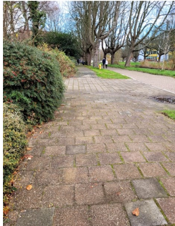
Figure 24: Sidewalk pavers test area for strollers. ALT TEXT: Photo of sidewalk pavers for strollers.
