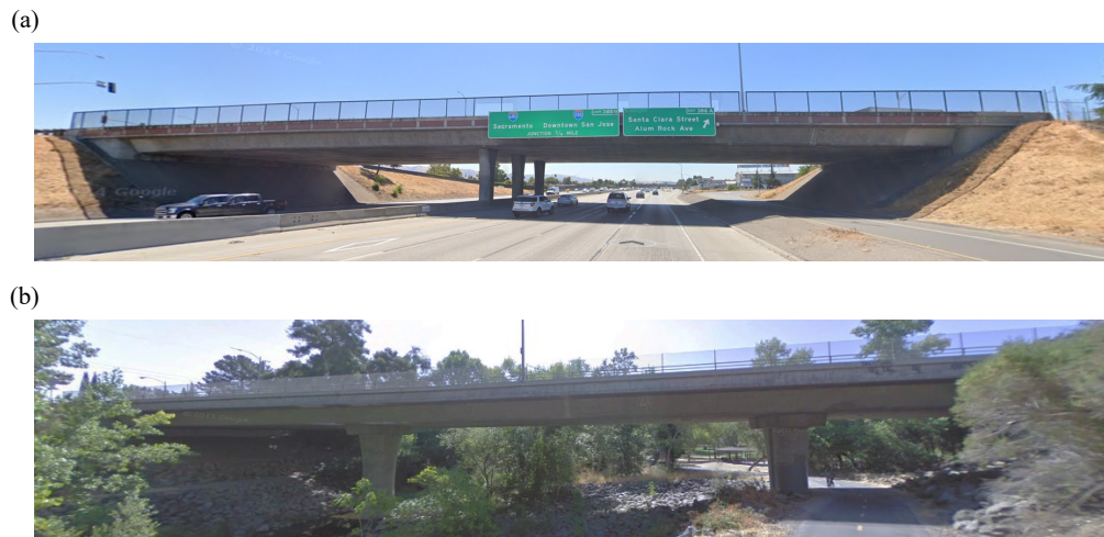
Figure 4: Street view images (Google Maps) of (a) Bridge 1, McKee Road over U.S. Highway 101 Overpass and (b) Bridge 2, Yerba Buena Road over Coyote Creek Bridge.
