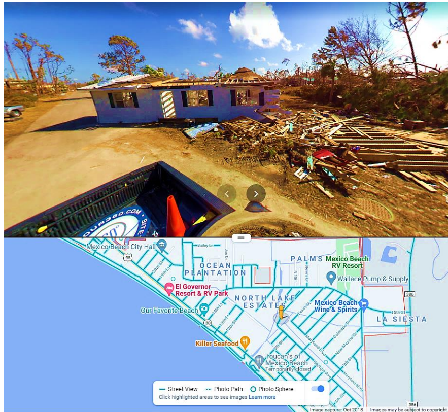
Figure 14. Post-event imagery of Mexico Beach following Hurricane Michael (October 10, 2018) illustrating observed structural damage for validation purposes.
