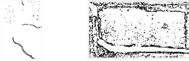
(a) Cracks on plain concrete (b) Cracks on brick surface
