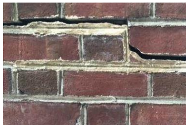
Fig. 16: Crack between bricks
