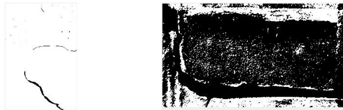
(a) Cracks on plain concrete
