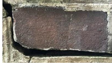
(b) Cracks on brick surfaces
