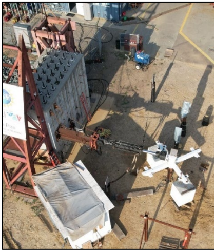
c) Pile Test 01 – Post Test Layout
