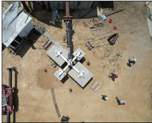
d) Direct overview of Test Pile 04
