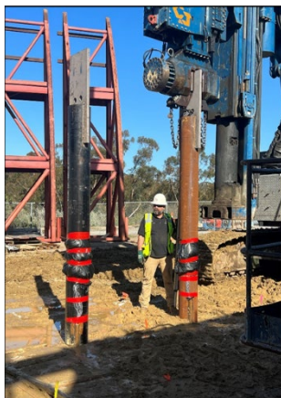
a) Pile Installation D/t 22 & D/t 43 (b) Pile Installation Pile #2 with Vibratory Hammer
