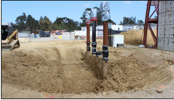
(a) Soil Pit Excavation – Day 1
