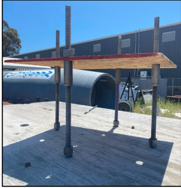
(a) Concrete Block Anchorage Installation
