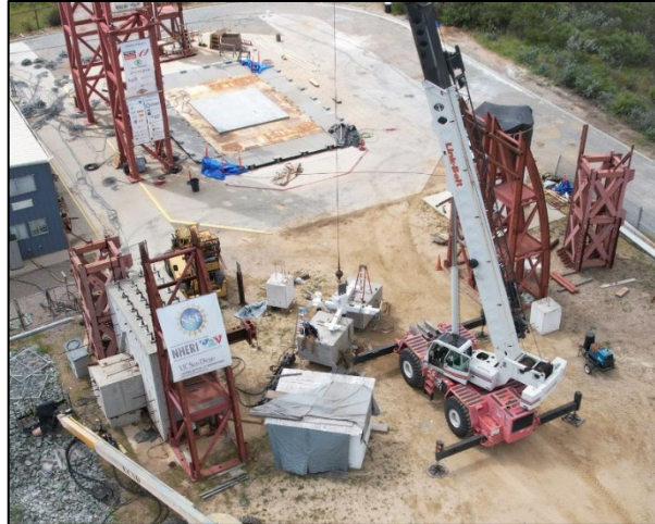
b) Pile Test 03 Set up in April 2024
