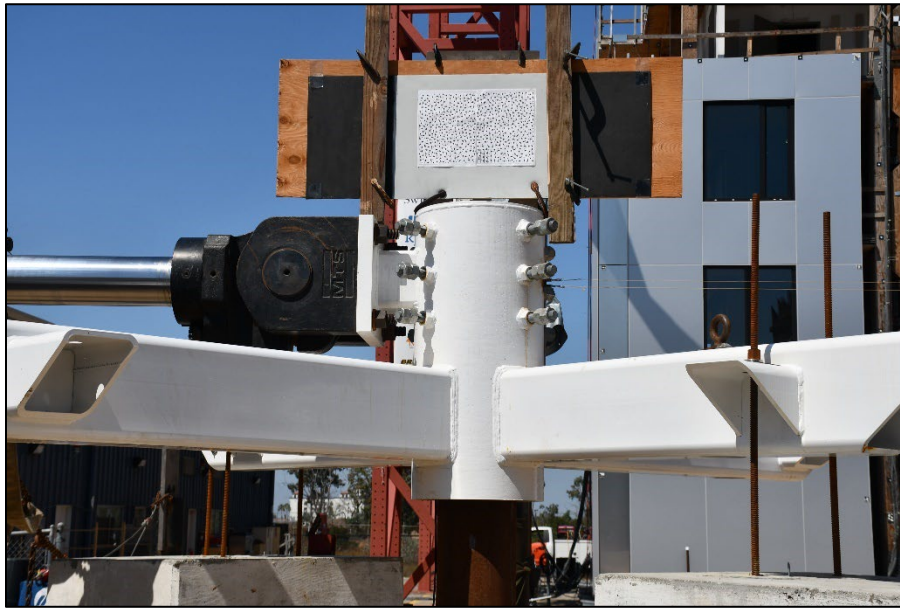
Figure 22: Top of Pile DIC Instrumentation
