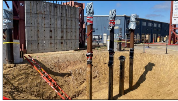
(b) Final Soil Pit Excavation
