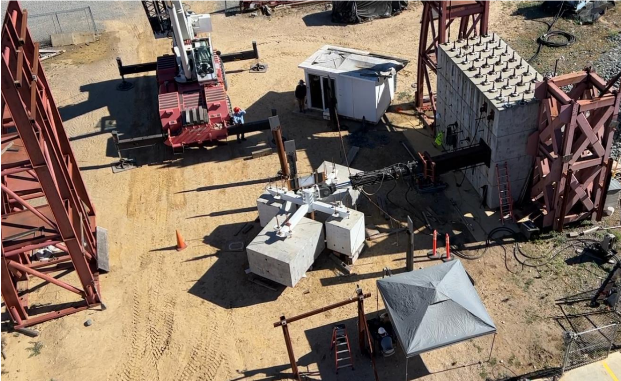
Figure 3: Overview Pile Test Set-Up
