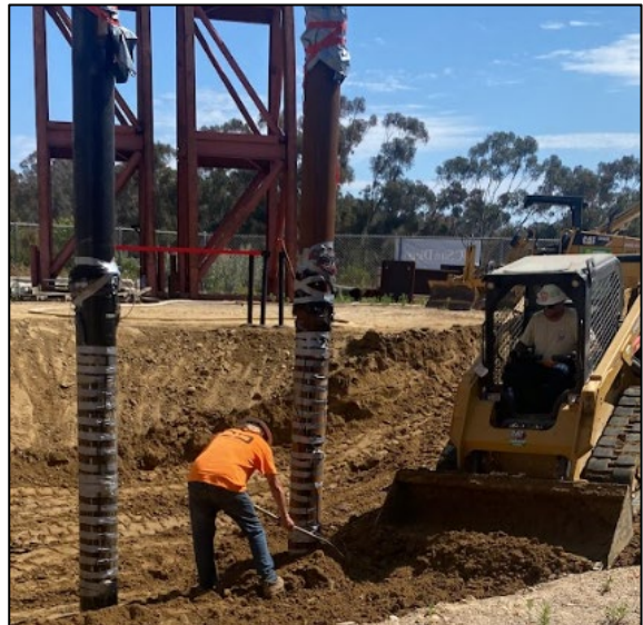
(e) Backfill Soil Pit
