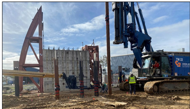
a) Pile Installation D/t 22 & D/t 43 (b) Pile Installation Pile #2 with Vibratory Hammer
