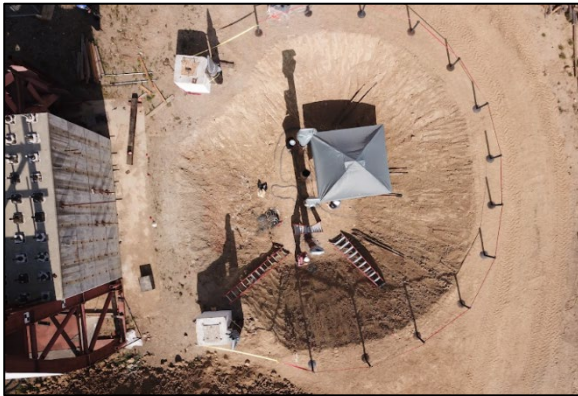
(c) Soil Pit Excavation Overview
